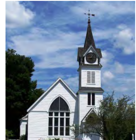
Second Congregational Church, Jeffersonville
