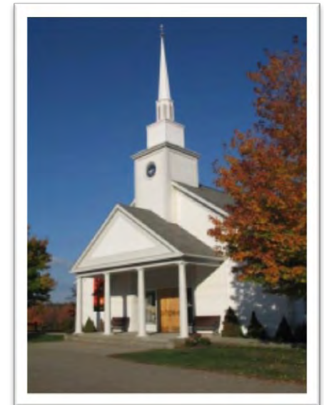
Malletts Bay Congregational Church, Colchester
